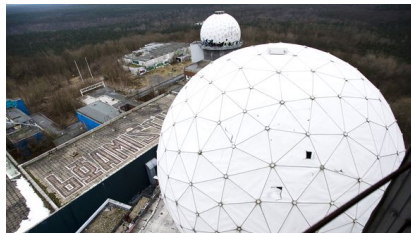
Former US listening station at Teufelsberg, Berlin.
